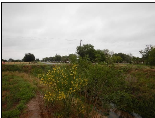
Photograph 63 – View looking northeast (downstream) at the existing Raymondville Drain and an adjacent residential area located near Lasara.
