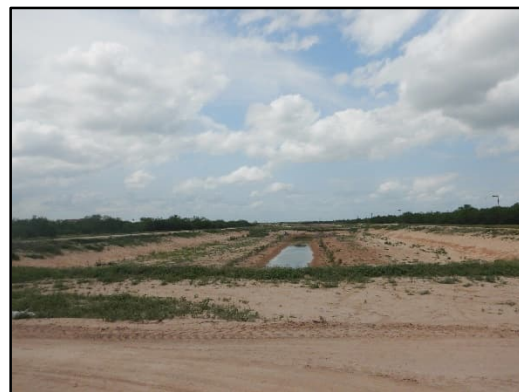
Photograph 6 – View looking further north than Photograph 4.
