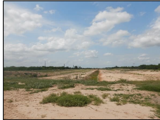
Photograph 4 – View looking further north than Photograph 2.
