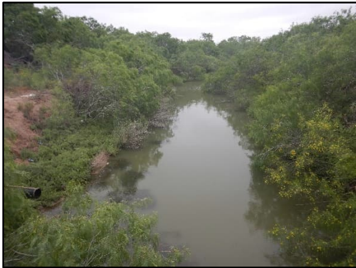
Photograph 37 – View looking east (downstream) at the existing Raymondville Drain.
