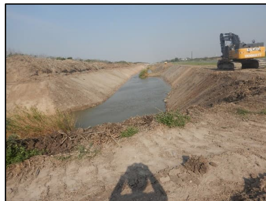
Photograph 90 – View looking east (downstream) at the existing Raymondville Drain near US 77.
