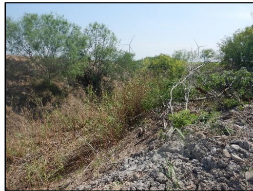
Photograph 95 – View looking south at a vegetated drainageway which flows into the existing Raymondville Drain.
